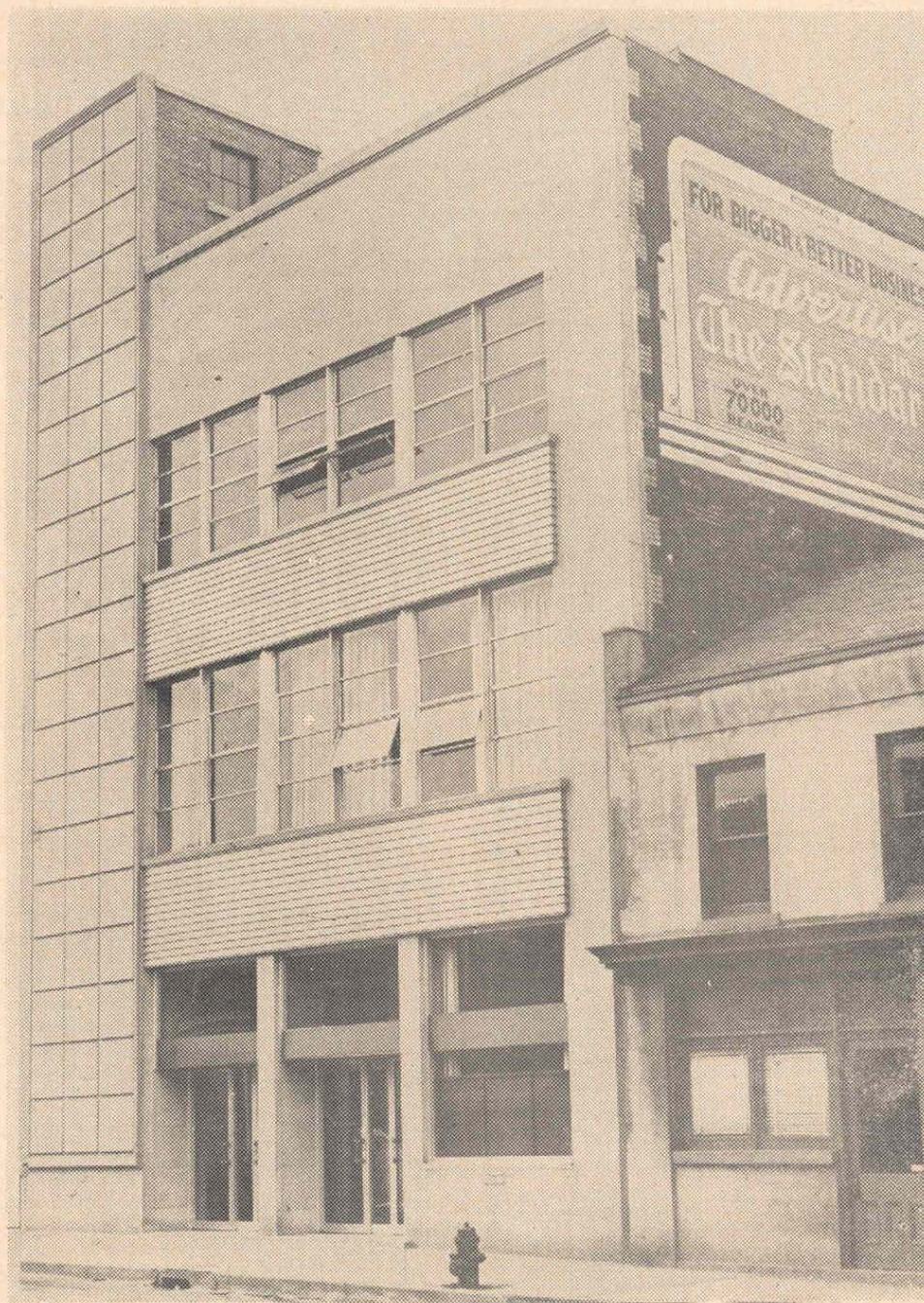
Newly Renovated Offices of "The Standard"
